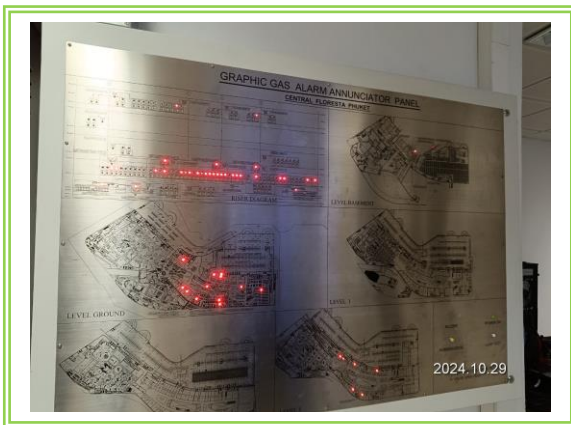
Graphic Annunciator Fire Protection System
